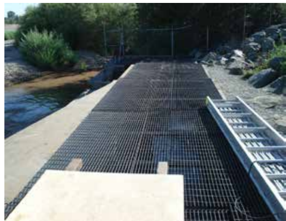
Figure V-a. Installation of metal grates on the Daguerre Point Dam fish ladder bays during August 2011 (from biological assessment).
