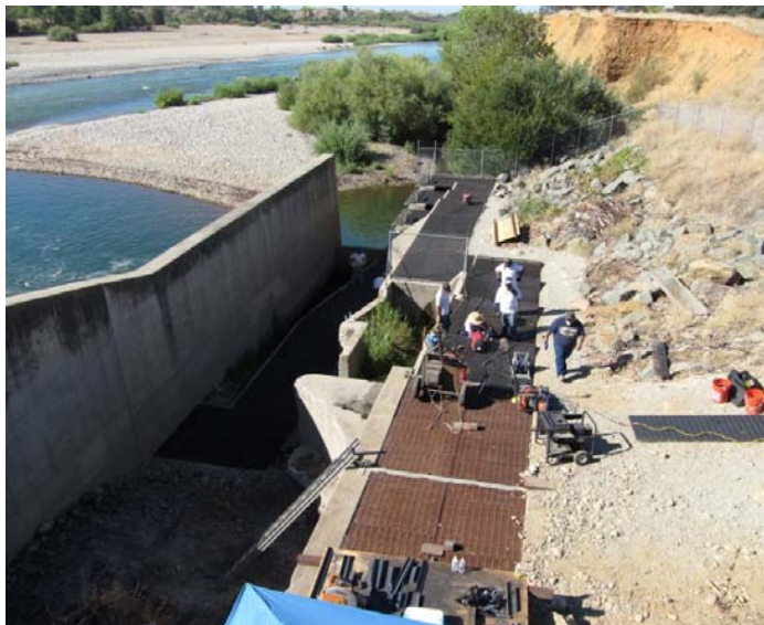
Figure 5-1. Installation of metal grates on the Daguerre Point Dam fish ladder bays during August 2011 (Corps 2011).
