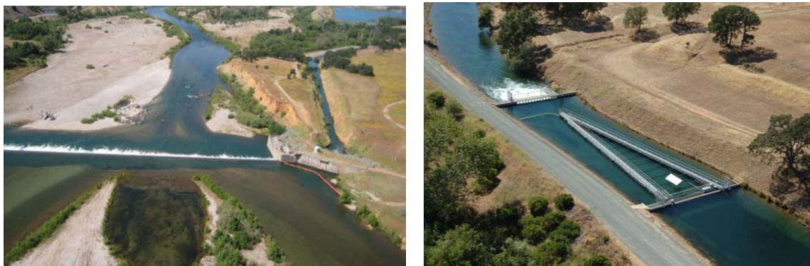
Figure 5-5. Hallwood-Cordua Diversion. Image on the left shows the control gate headworks on the north abutment of Daguerre Point Dam. Image on the right shows the current v-shaped screen (Source: YCWA 2013b).
