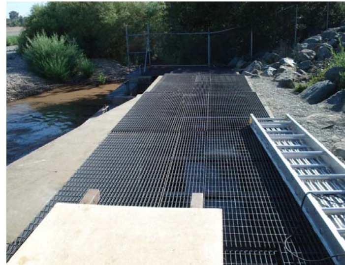
Figure 5-1. Installation of metal grates on the Daguerre Point Dam fish ladder bays during August 2011 (Corps 2011).
