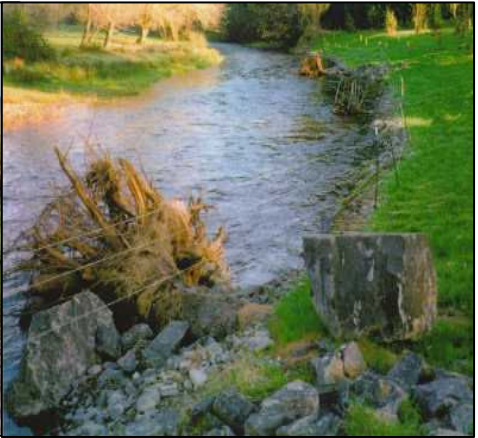
Photo 28: Cedar Creek After - stable revegetated banks and root wads.
