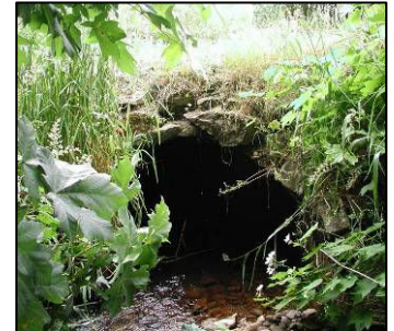
Photo 30: Jackson Creek before culvert replacement.
