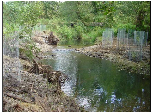
Photo 34: South Fork Chelatchie Creek After two deep new pools with root wads, vanes, and spawning beds.
