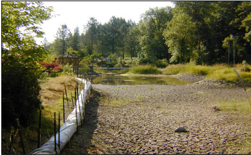
Photo 7: Manly Road Creek Before - old man-made pond in middle of creek leaking flow and drying up.
