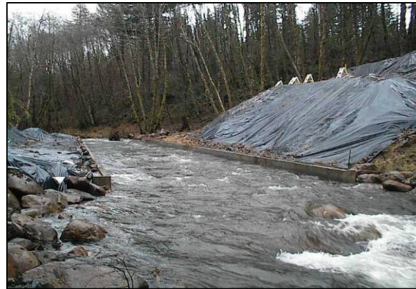
Photo 27: Cedar Creek In Progress - streambed prior to domed culvert placement.
