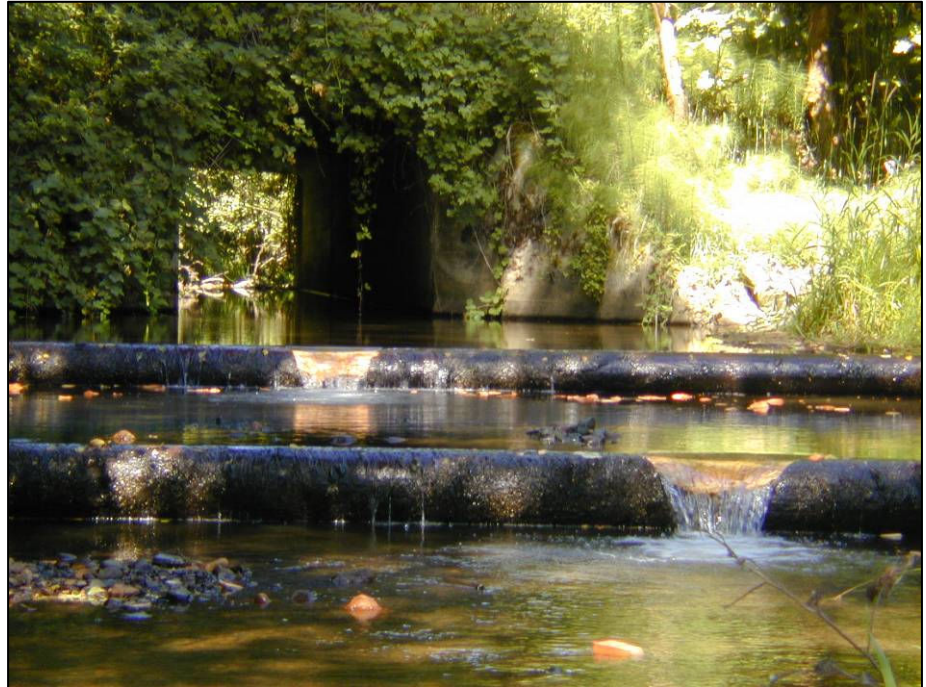
Photo 4: Lockwood Creek After - check dam modification for fish passage improvement.
