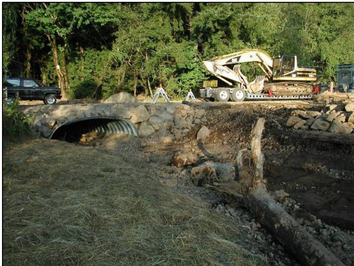
Photo 31: Jackson Creek After new culvert placement.
