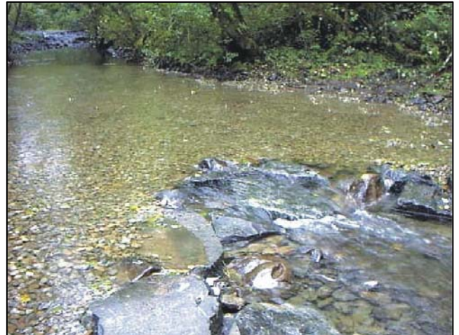
Photo 19: Cedar Creek After - in-stream cross-vane with spawning gravel added above.
