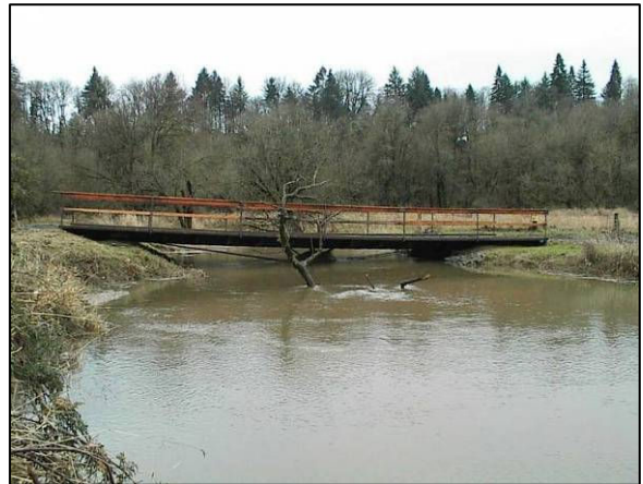
Photo 5: Lockwood Creek After - bridge replacing old culvert, restoring creek flow.
