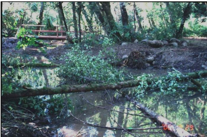
Photo 18: Cedar Creek After - new side channel rearing area with a juvenile fish viewing bridge.
