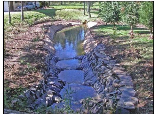
Photo 32: Cedar Creek Tributary After side channel, main pool, and step-pools leading to the spring above.
