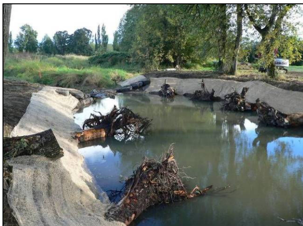
Photo 9: Mason Creek After - deep pool and root wad (LWD) cover and habitat.
