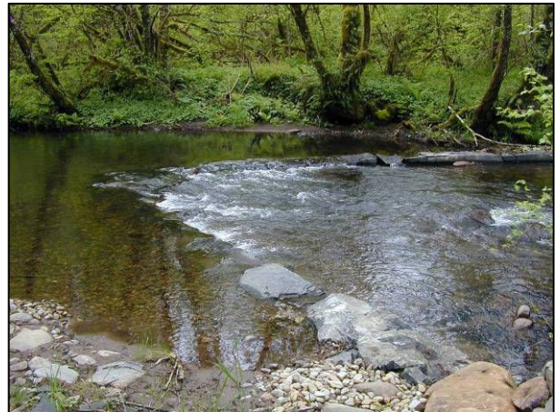
Photo 17: Cedar Creek After - cross vane with deep pool below and spawning gravel at head of vane along with LWD root wads.
