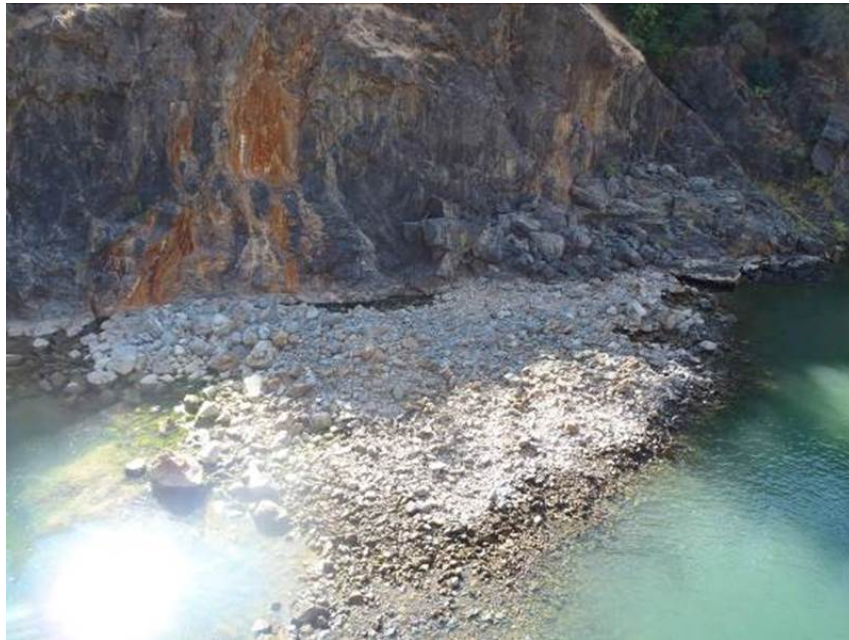
Figure 3.1-1. Picture of dry gravel bar on which the work would occur. The photo was taken during a Narrows 2 outage when no flow was being released from the Narrows 2 Facilities. 32
