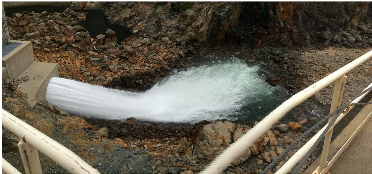
Figure 2.1-3. Operation of the Full Bypass at a discharge of 100 cfs on October 15, 2014.
