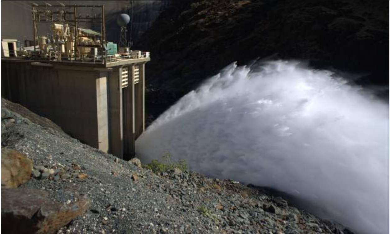
Figure 2.1-2. Operation of the Partial Bypass at Narrows 2 Powerhouse. The discharge through the Partial Bypass at the time this photo was taken is unknown.
