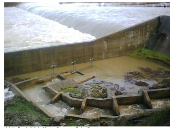
Figure 4.2-2. South fish ladder at Daguerre Point Dam.
