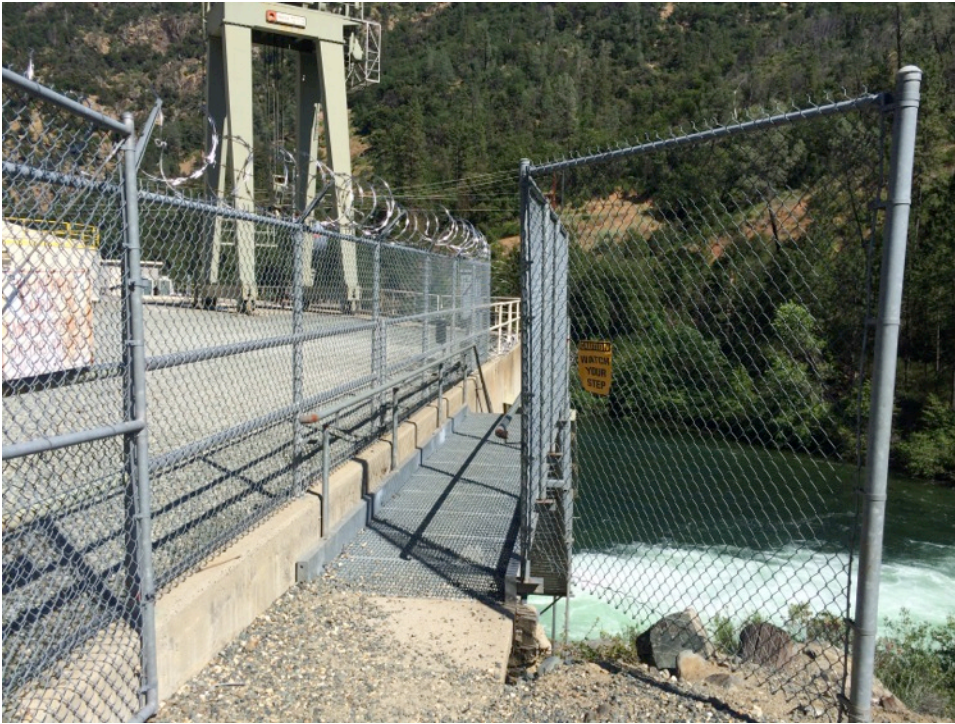
Figure 1, Existing Powerhouse Catwalk
