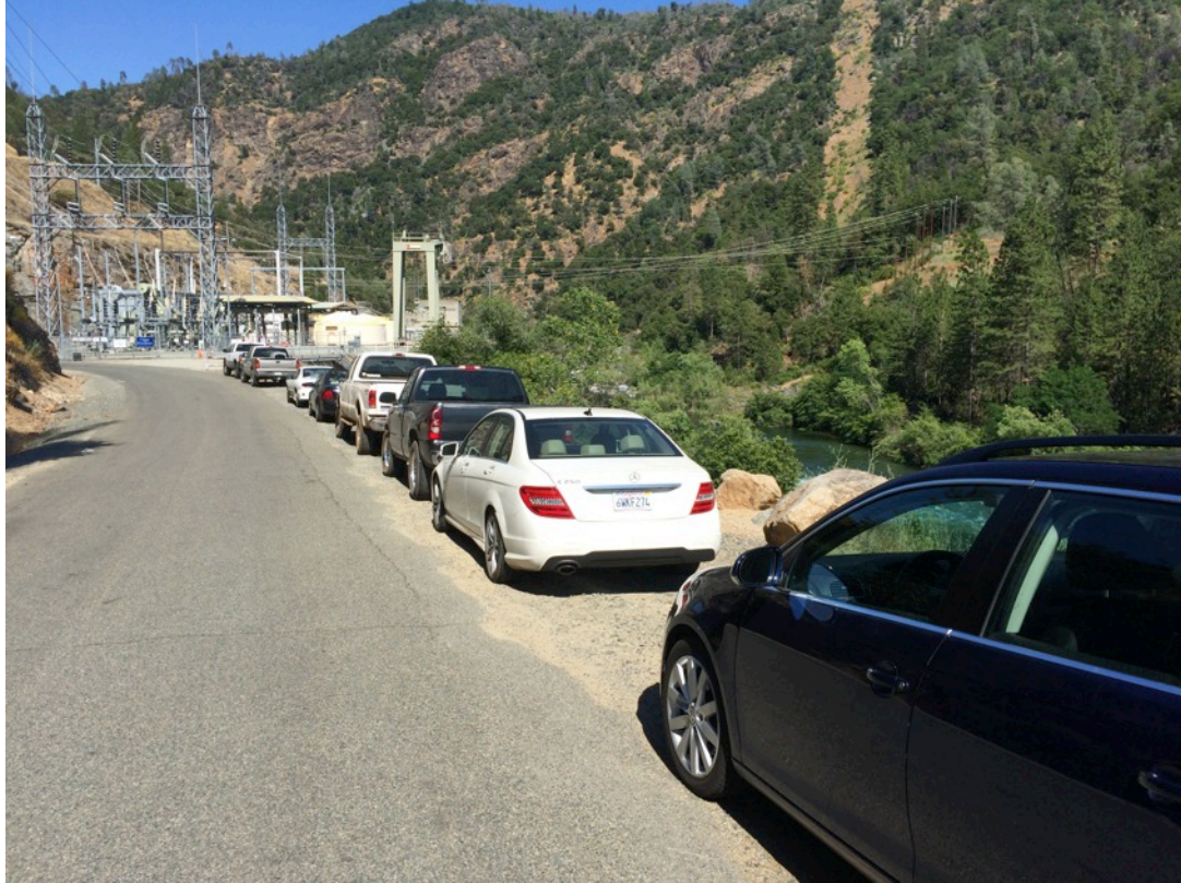
Figure 3, New Colgate Powerhouse Parking
