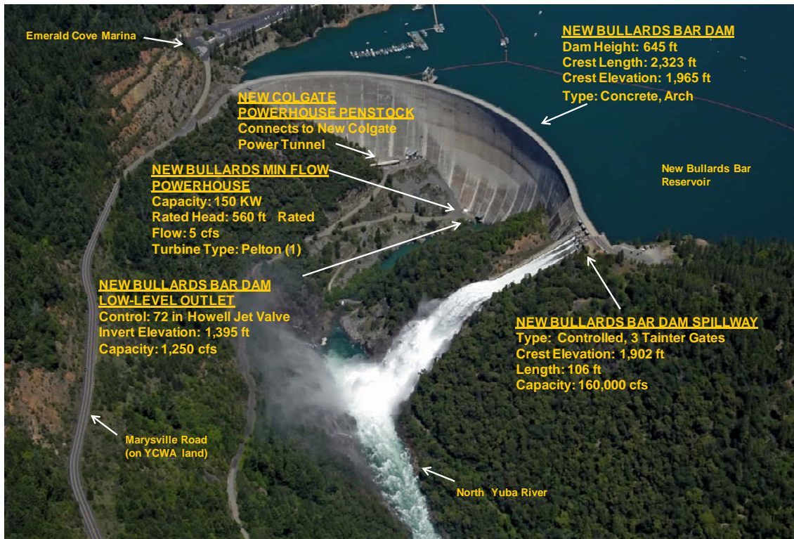
Photo 3. New Bullards Bar Dam and New Bullards Bar Minimum Flow Powerhouse.
