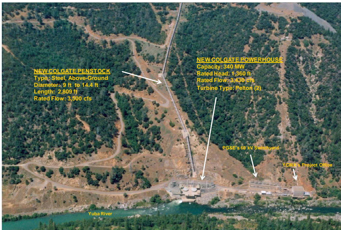
Photo 4. New Colgate Powerhouse and Penstock.
