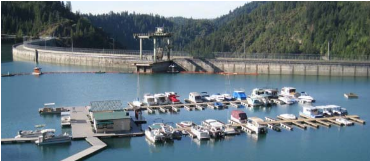
Figure 7.8.2-3. Photograph of Emerald Cove Marina including boat slips, floating store and fuel station (photo May 12, 2009).
