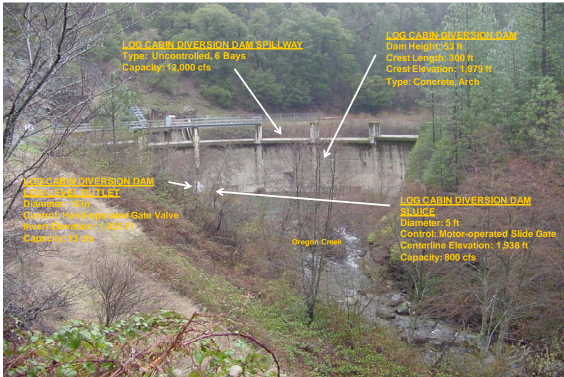
Photo 2. Log Cabin Diversion Dam.
