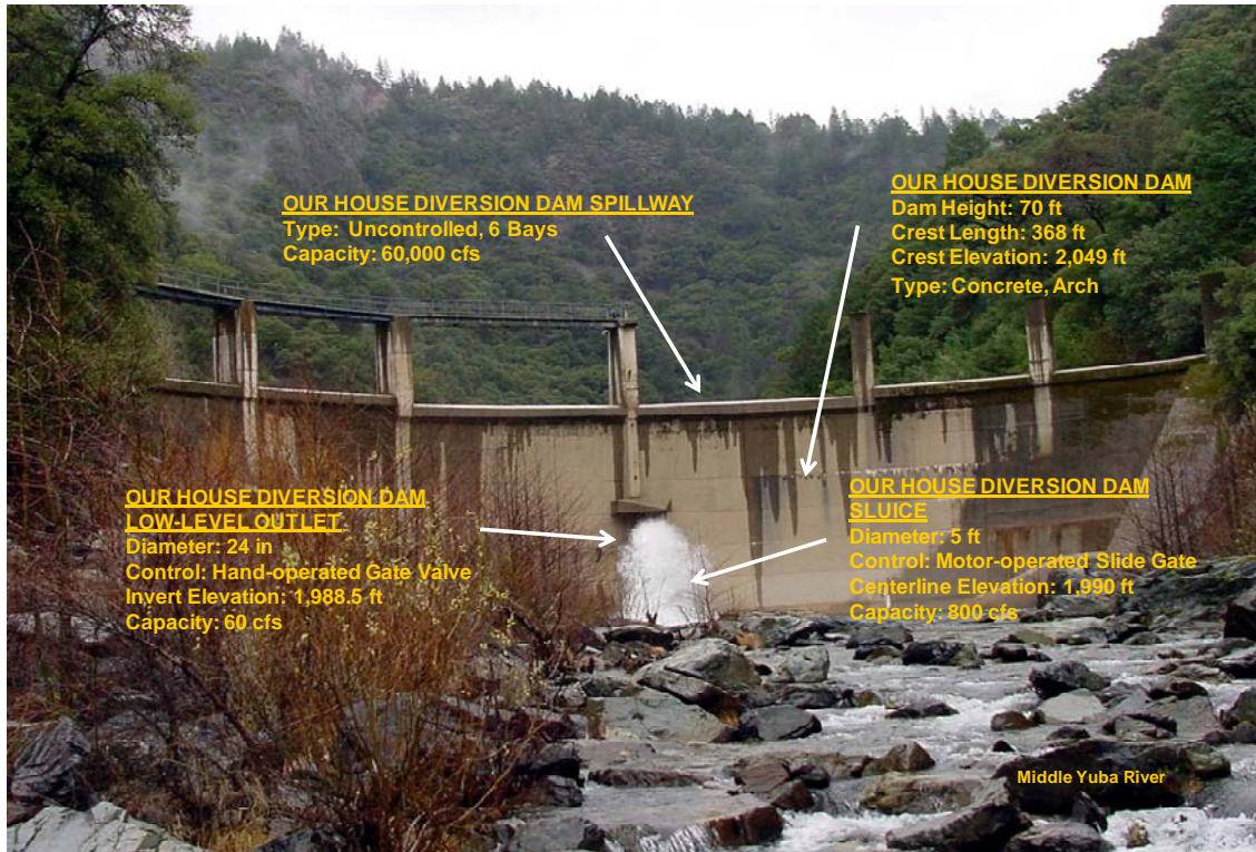
Photo 1. Our House Diversion Dam.
