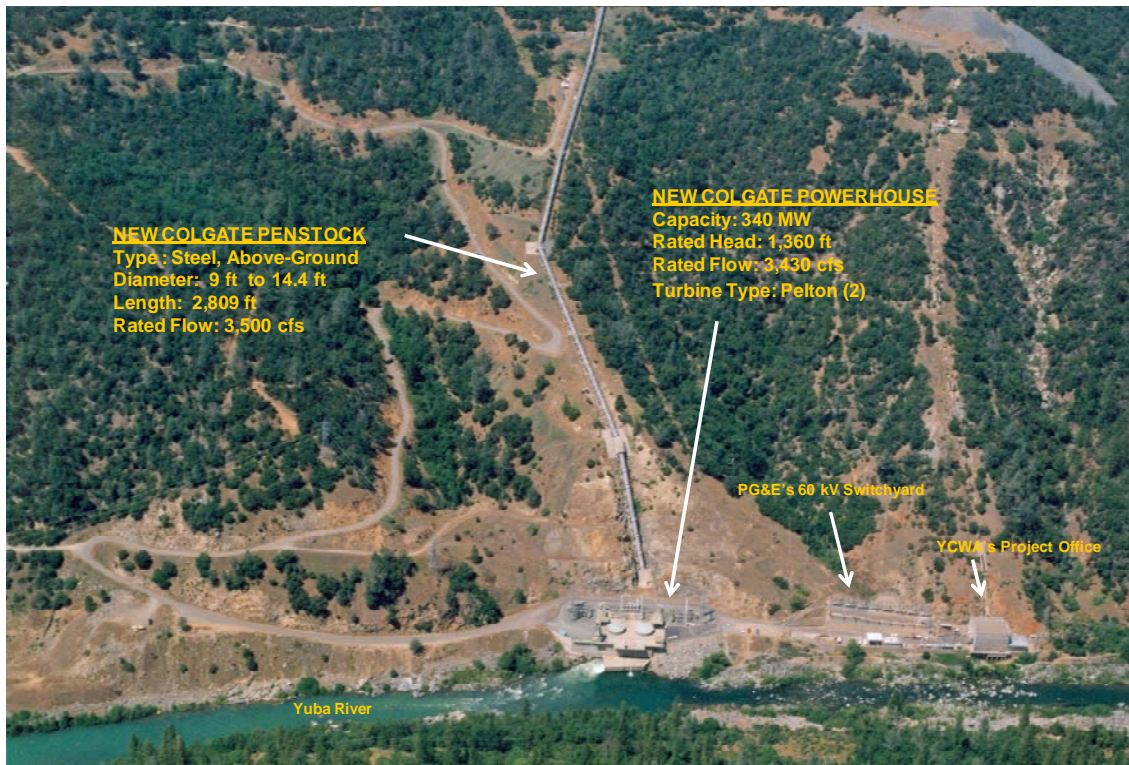
Photo 4. New Colgate Powerhouse and Penstock.
