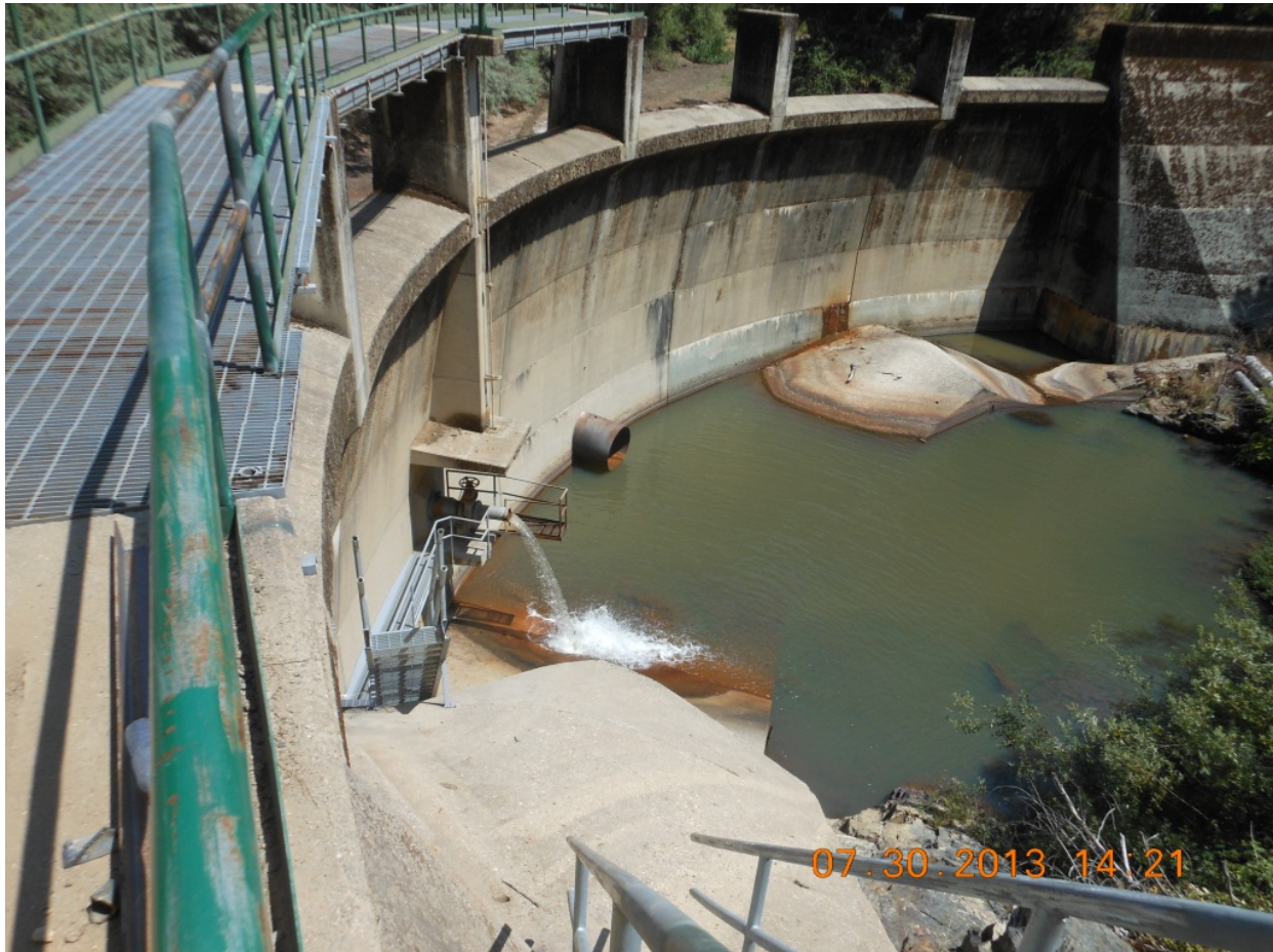
Figure 2.2-1. View to the east of the downstream face of Log Cabin Diversion Dam. The majority of discharge is through the fish release valve. The low level outlet valve is to the right of the fish release valve.
