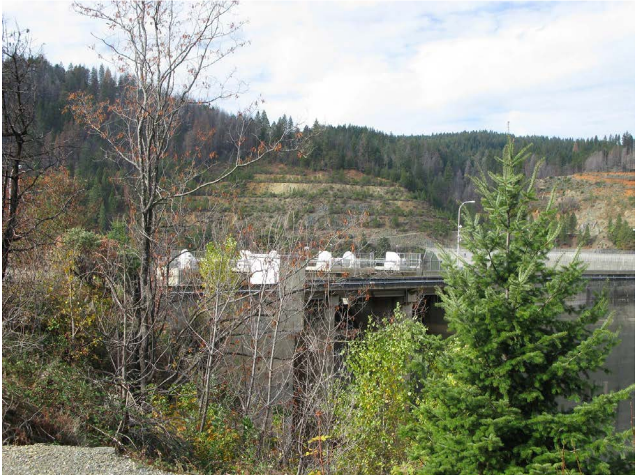
Figure 3.2-1. Photograph of the New Bullards Bar Dam gate controls and housings.
