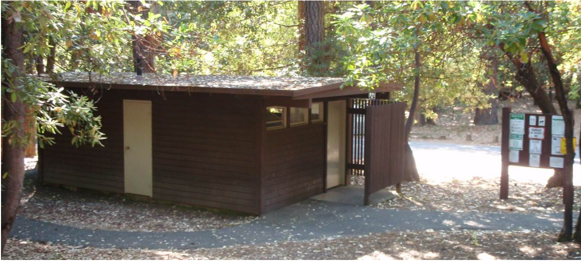
Typical Comfort Station
