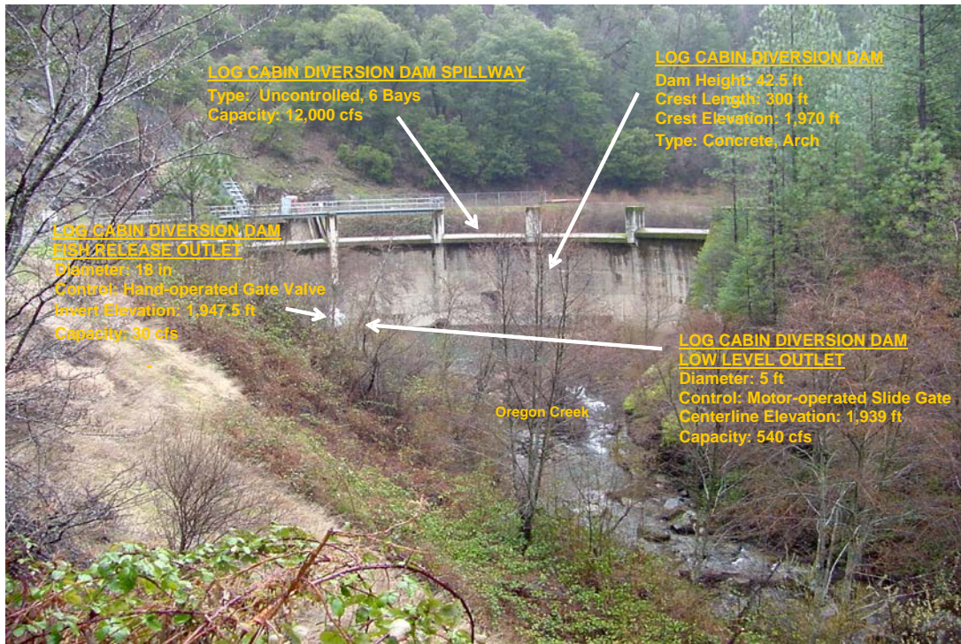
Figure 3.1-2. Log Cabin Diversion Dam.
