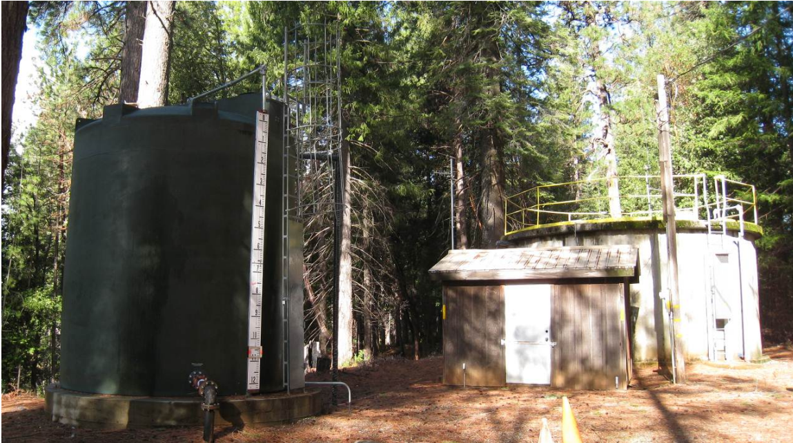
Figure 3.1-21. Representative photograph of the water storage tanks.
