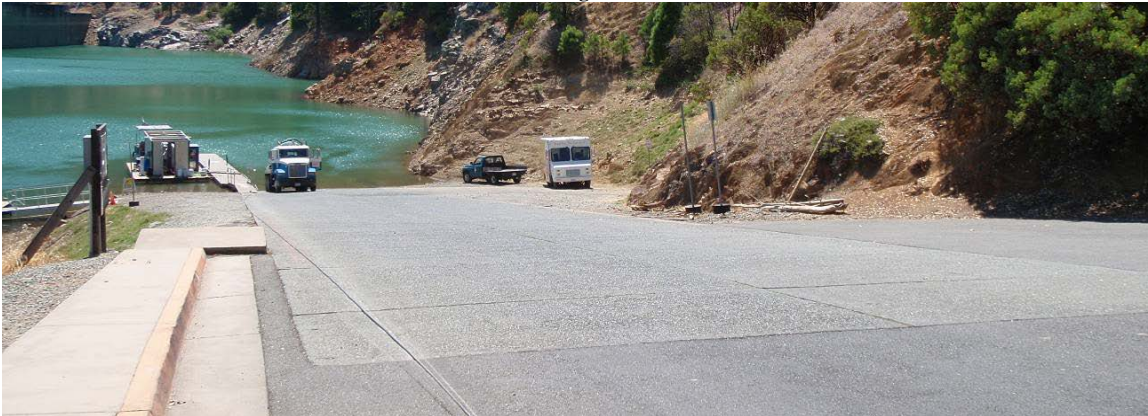
Boat Ramp and Floating Dock
