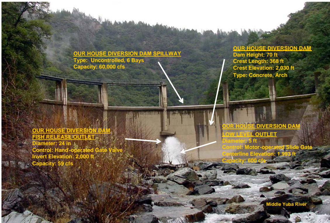
Figure 3.1-1. Our House Diversion Dam.
