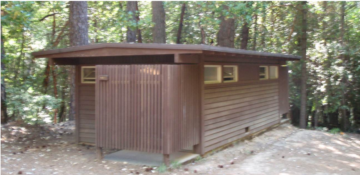
Typical Comfort Station
