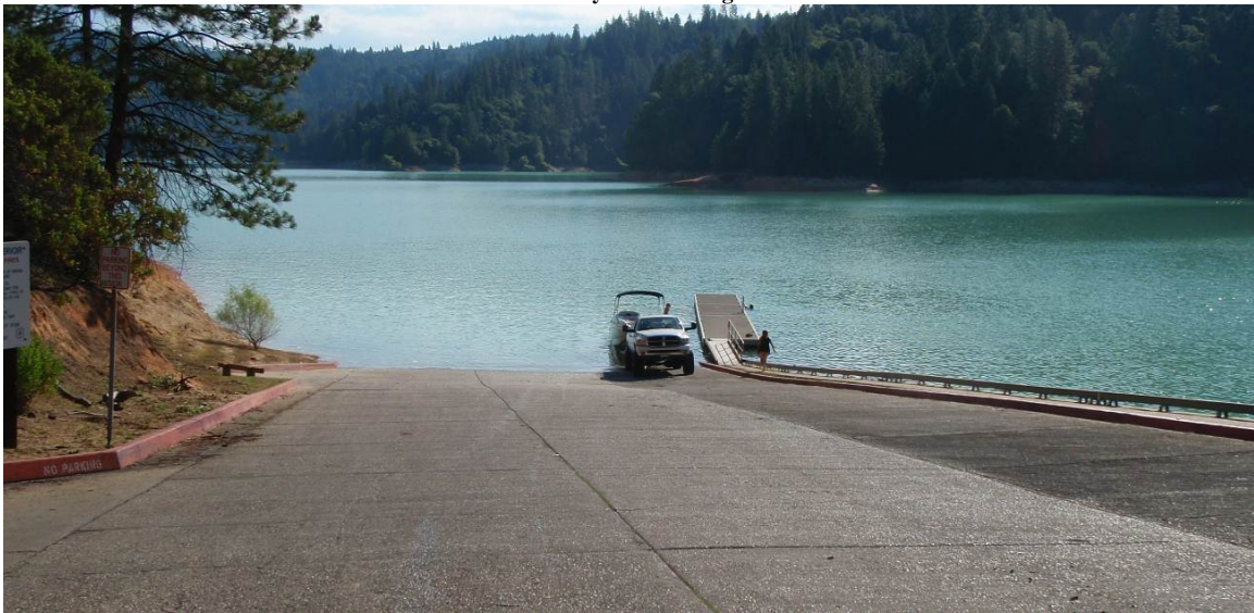
Boat Ramp and Floating Dock
