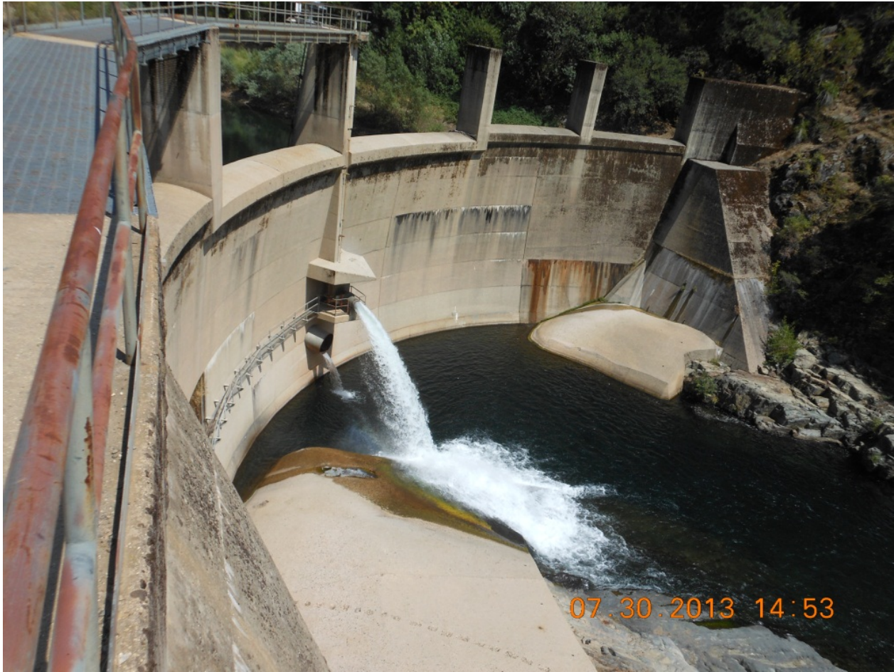
Figure 2.2-1. View to east of downstream face of Our House Diversion Dam. The majority of discharge shown in photograph is through the fish release valve. A minor amount of gate leakage is occurring through the low level outlet valve, which is below the minimum flow release valve.
