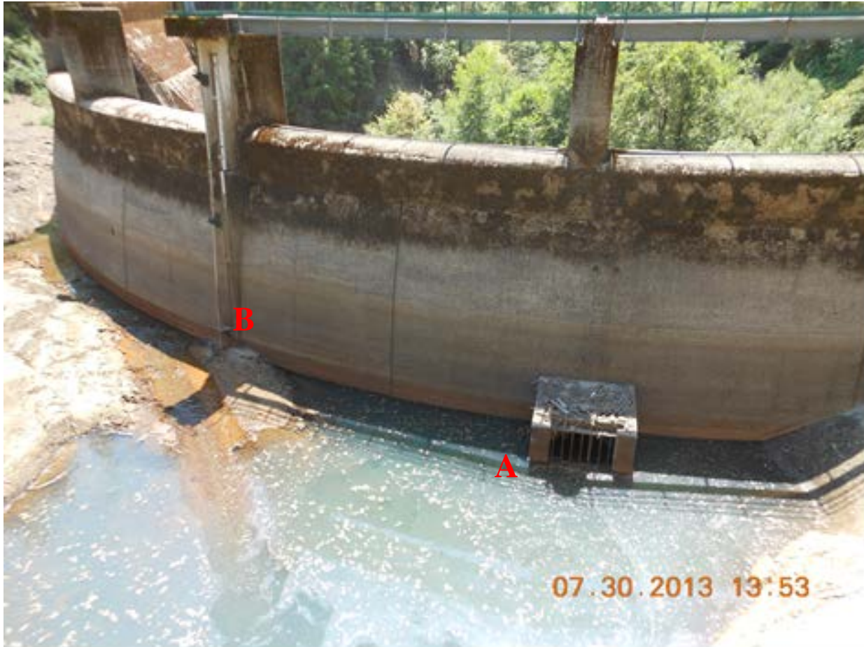
Figure 2.1-2. View to southwest of the upstream face of Log Cabin Diversion Dam. The intake for the fish release valve is marked by an “A;” the location of the intake valve stem for the low level valve is marked with a “B.”
