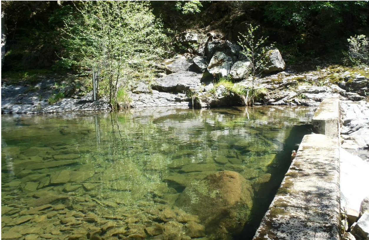
Figure 3.1-3. Oregon Creek downstream Log Cabin measurement weir, weir box, and gage pool.
