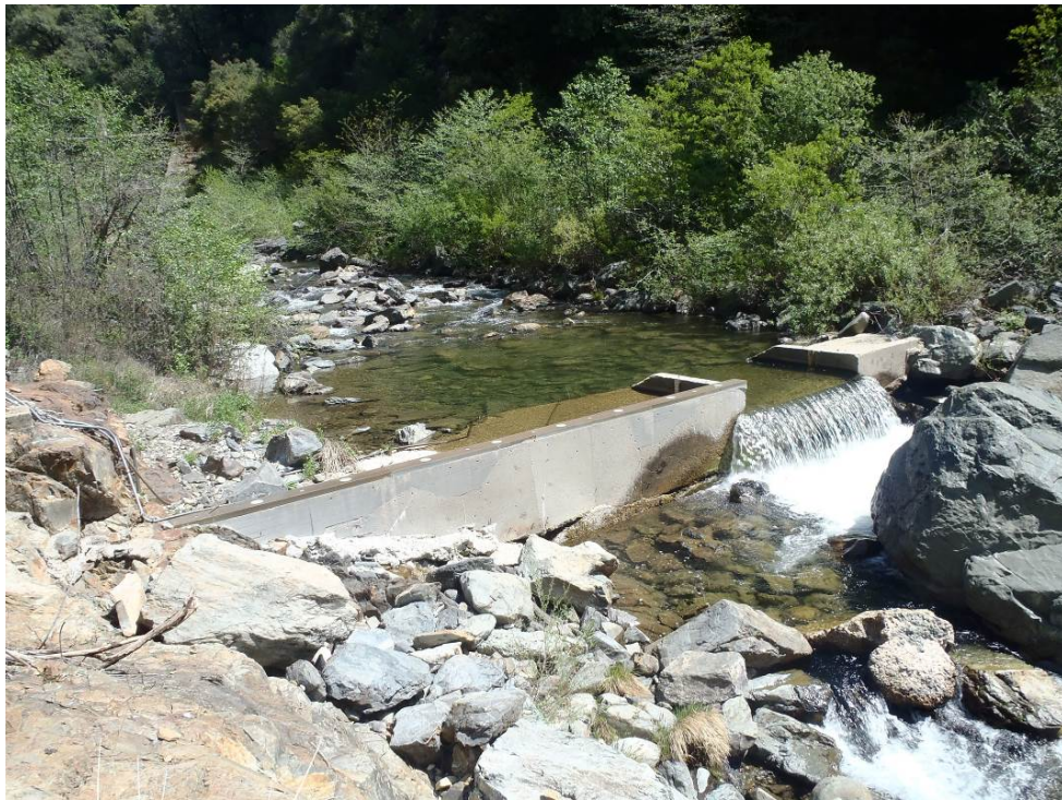
Figure 3.1-2. Middle Yuba downstream from Our House Diversion Dam gage pool and sharp-crested weir.
