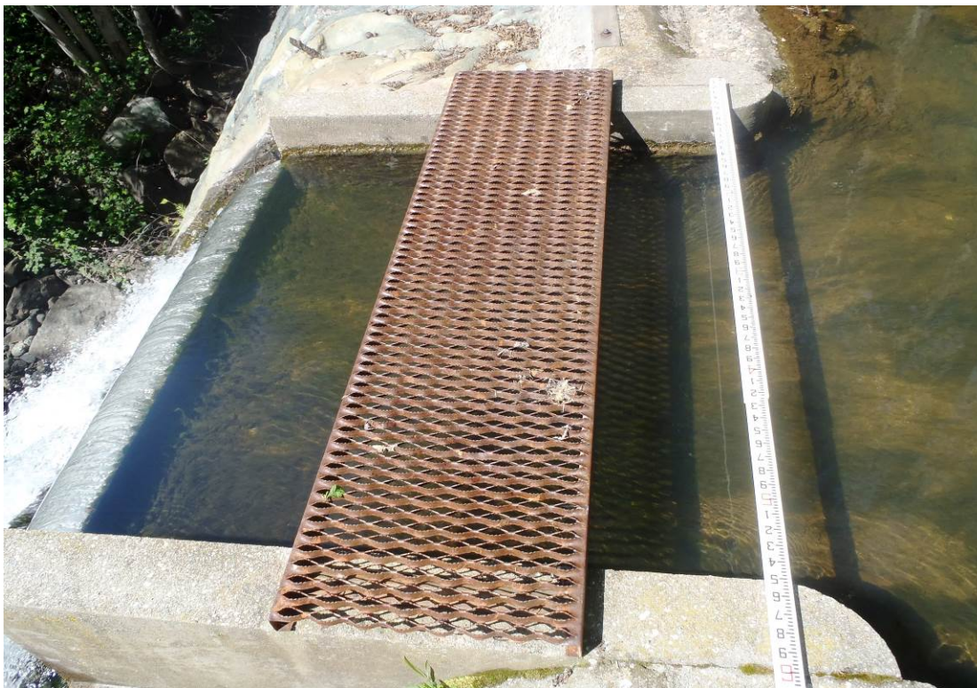
Figure 3.1-5. North Yuba River downstream from New Bullards Bar Dam flow measurement weir box.
