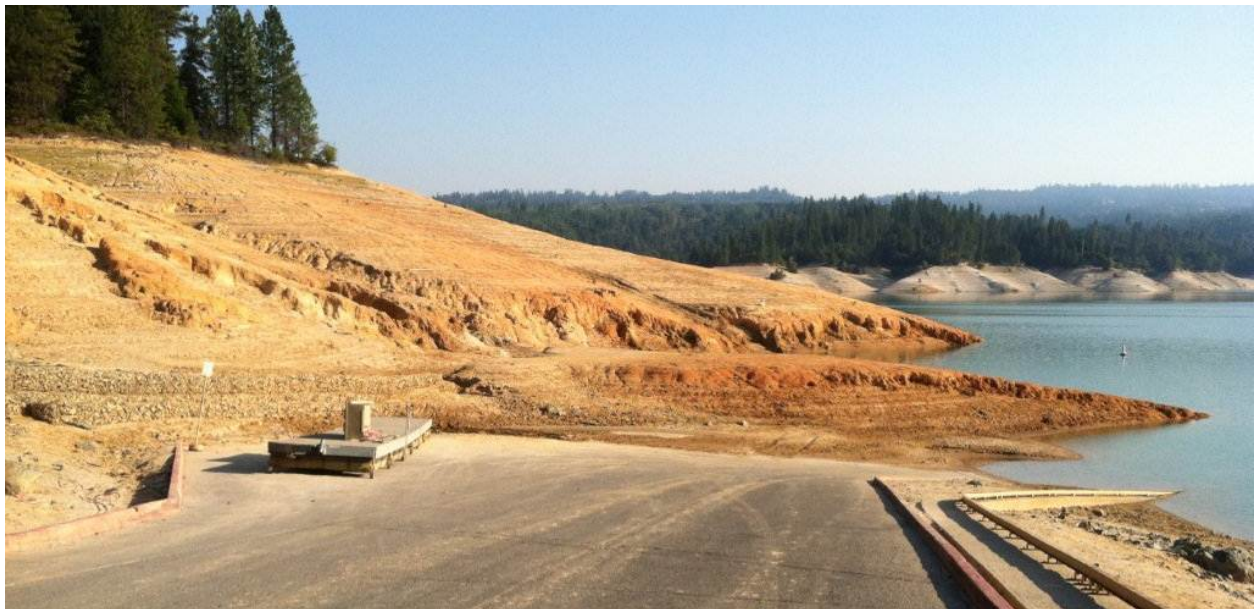
Figure 3.3.6-2. Photograph of the slope instability site upslope from the Dark Day boat ramp at low water levels (typically during the non-peak season). 23
