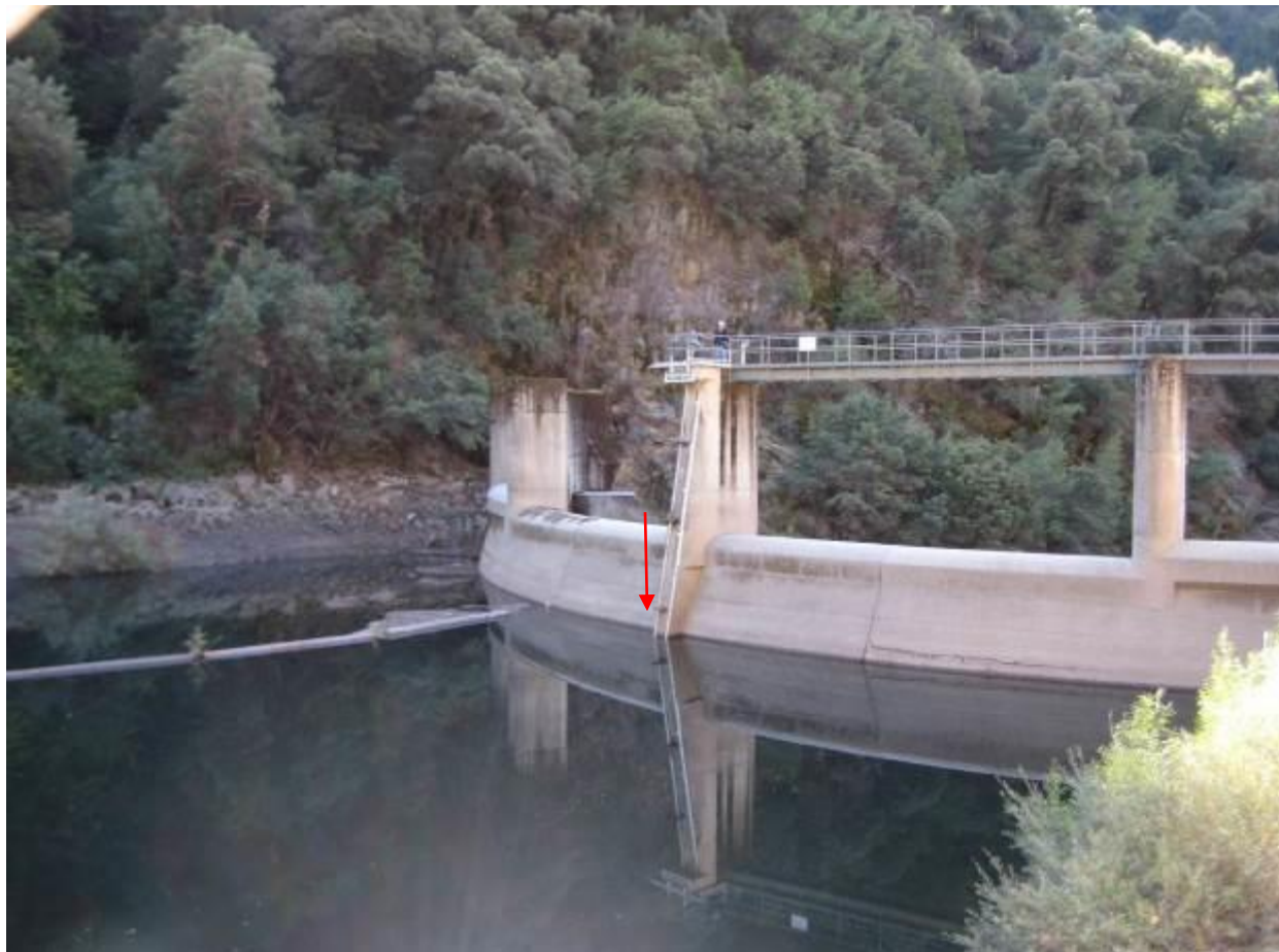
Figure 2.2-2. View to the south of upstream face of Our House Diversion Dam. The inlets for the low level valve and the fish release valve are located below the operator for the Low Level Valve, as indicated by the arrow above.
