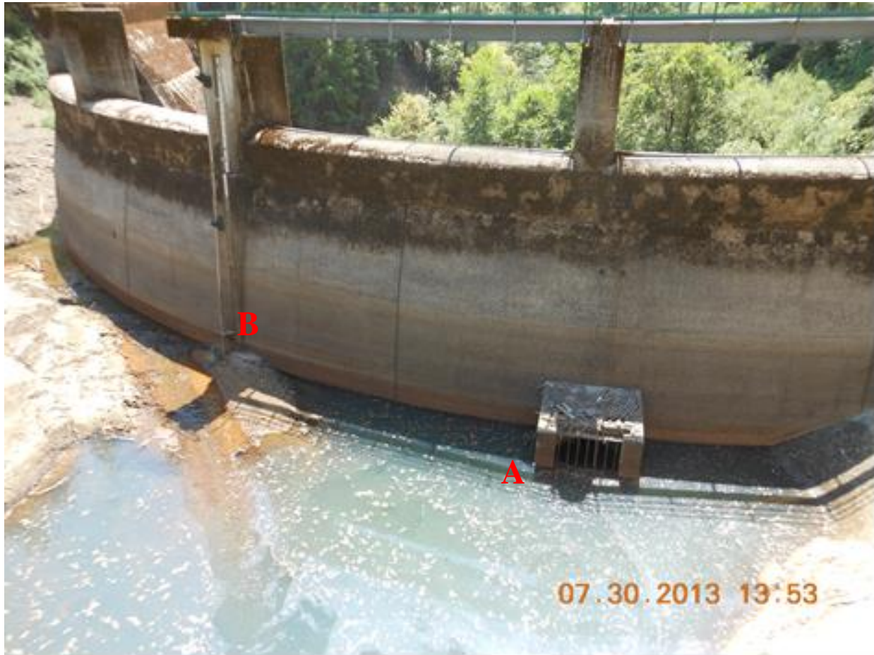
Figure 2.1-2. View to southwest of the upstream face of Log Cabin Diversion Dam. The intake for the fish release valve is marked by an “A;” the location of the intake valve stem for the low level valve is marked with a “B.”
