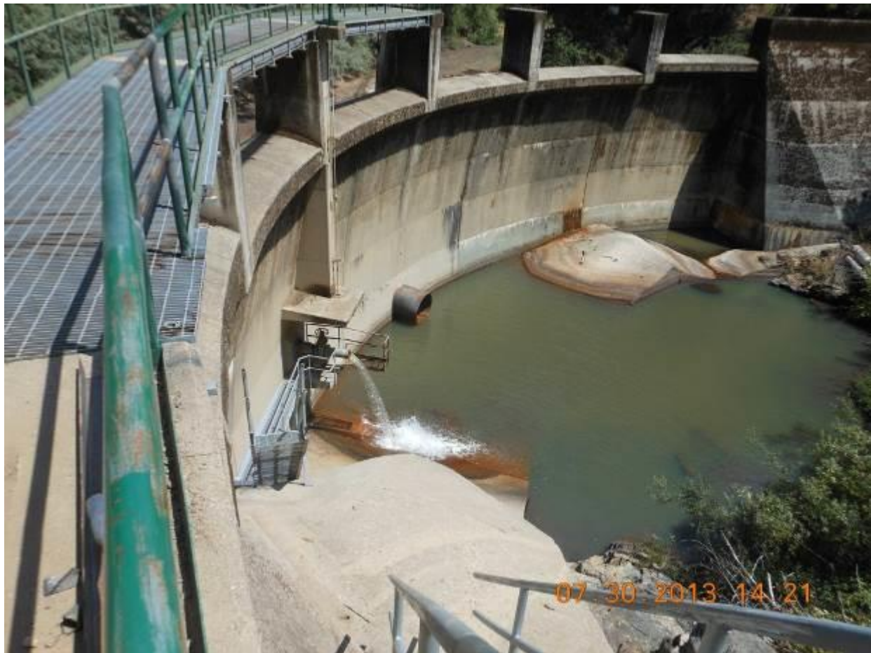
Figure 2.1-1. View to the east of the downstream face of Log Cabin Diversion Dam. The majority of discharge shown in photograph is through the fish release valve. The low level outlet valve is to the right of the fish release valve.
