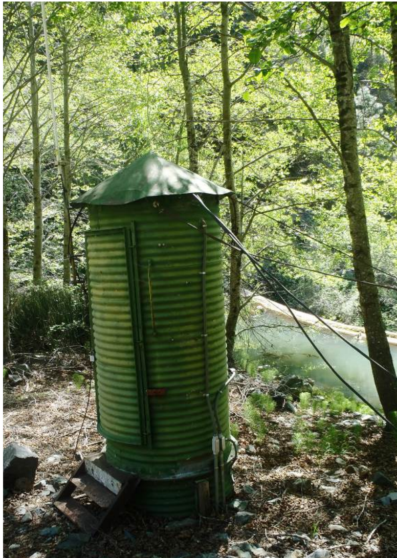
Figure 3.1-4. North Yuba River downstream from New Bullards Bar Dam gage shelter.
