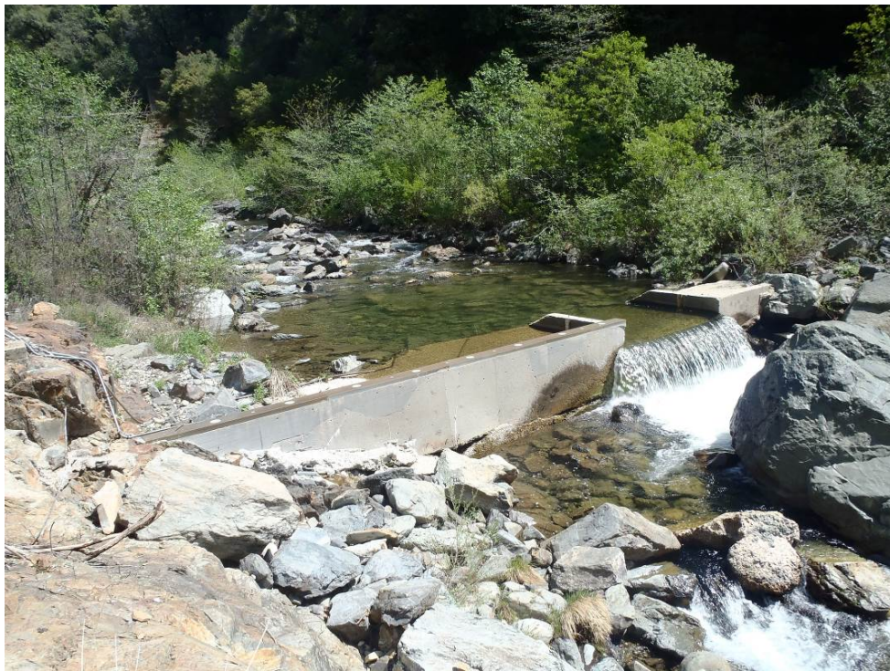
Figure 3.1-2. Middle Yuba downstream from Our House Diversion Dam gage pool and sharp-crested weir.
