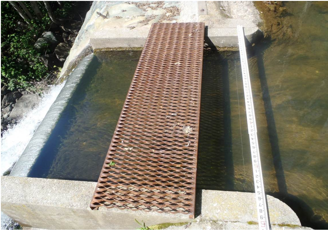
Figure 3.1-5. North Yuba River downstream from New Bullards Bar Dam flow measurement weir box.
