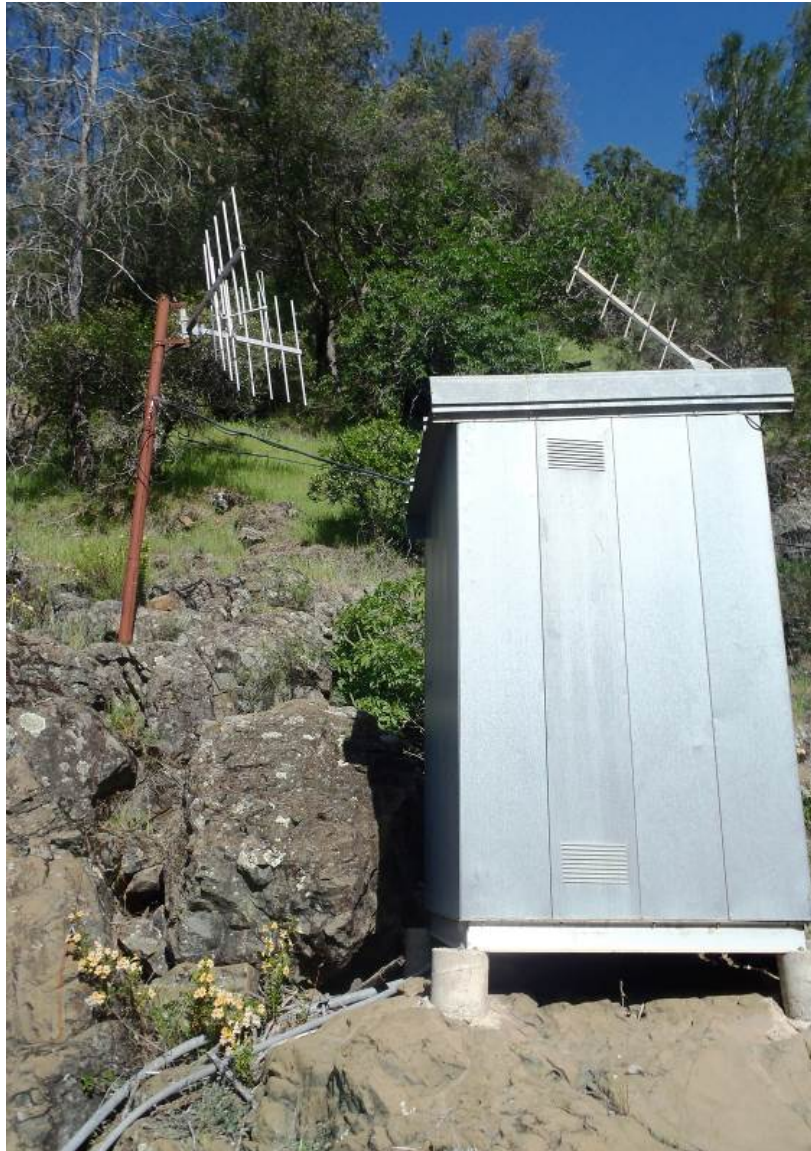
Figure 3.1-6. Yuba River downstream from Narrows 2 Powerhouse – Smartsville gage shelter.
