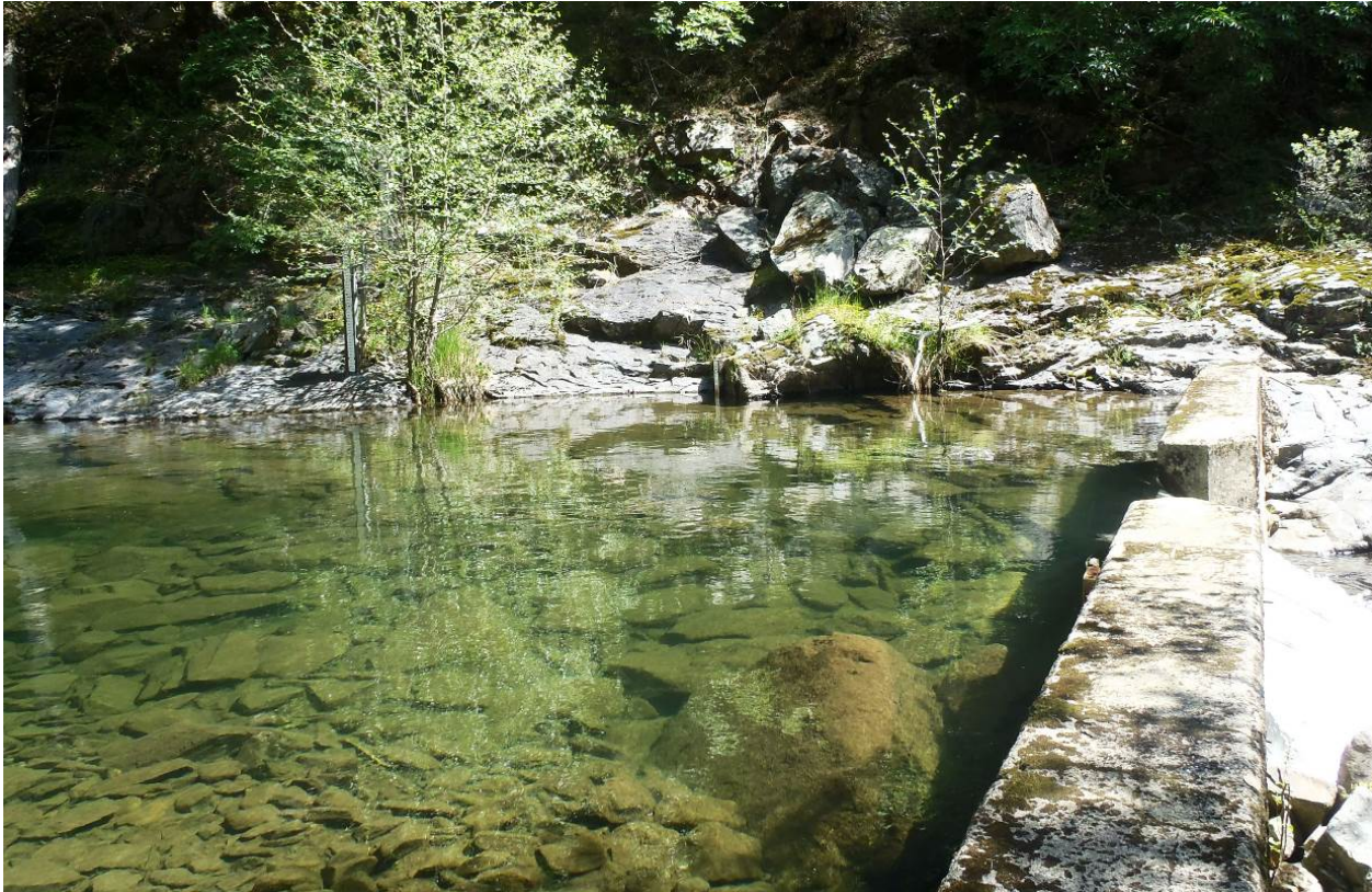
Figure 3.1-3. Oregon Creek downstream Log Cabin measurement weir, weir box, and gage pool.
