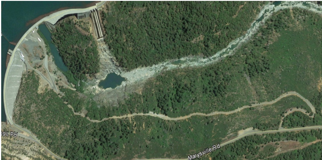
Figure 13. 2011 Google Earth© image showing YCWA’s access road from Marysville Road to New Bullards Bar Dam Dam and the spillway channel entering the North Yuba River.
