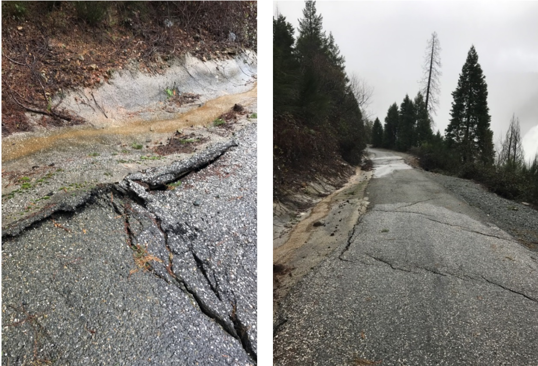
Figure 15. Photographs of Dam Access Road
