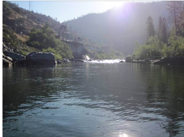
Figure 3.6-5. View from downstream at instream flow Transect 20 looking upstream to New Colgate Powerhouse outflow.
