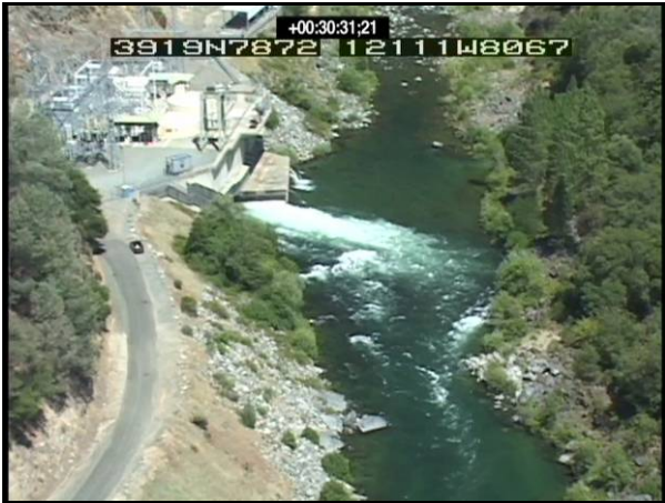
Figure 3.6-4. Aerial view of New Colgate Powerhouse outflow.
