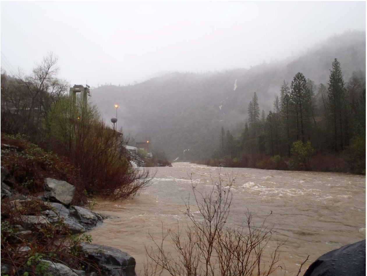
Figure 3.3-1. Yuba River looking upstream from below New Colgate Powerhouse on March 16, 2012. The powerhouse is on river left.
