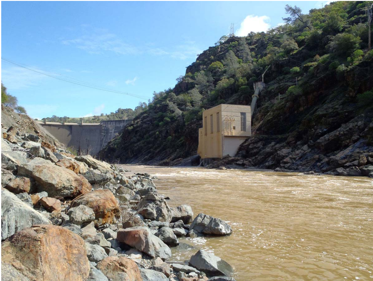
Figure 3.3-5. Yuba River below Narrows No. 1 Powerhouse on March 19, 2012. The powerhouse is on river right and Englebright Reservoir, which is not spilling, is in the background.
