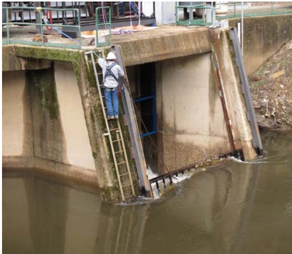
D) Blue antenna being cleaned after debris rack is removed.
