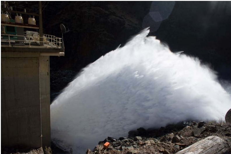
Figure 9. Narrows 2 Powerhouse during operation of partial bypass valve.
