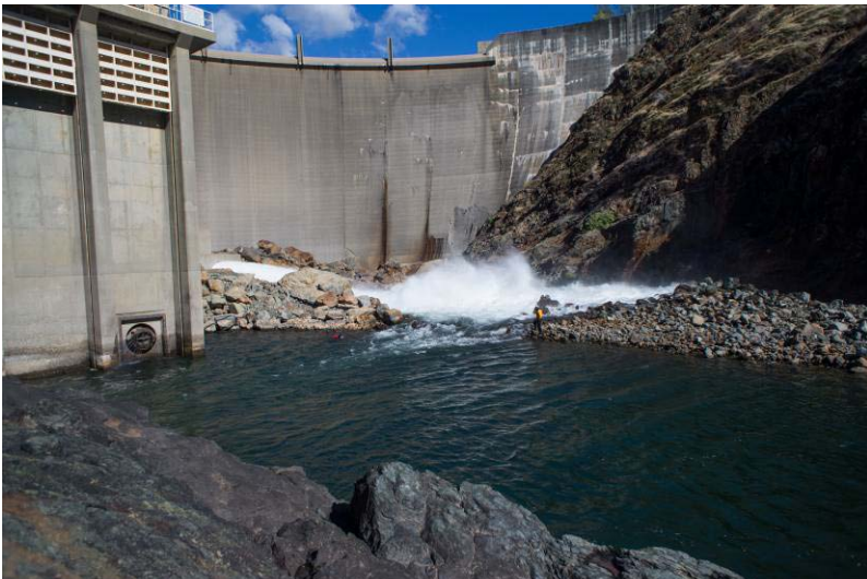
Figure 7. View of bypass pool (background) during operation of bypass valve.
