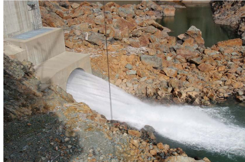
Figure 6. Operation of full bypass valve looking upstream from Narrows 2 Powerhouse.
