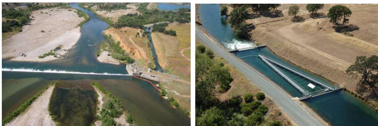
Figure 3.2-6. Hallwood-Cordua Diversion. Image on the left shows the control gate headworks on the north abutment of Daguerre Point Dam. Image on the right shows the current v-shaped screen.
