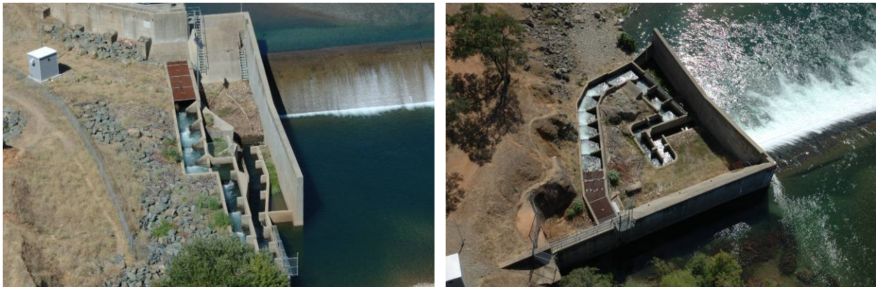
Figure 3.2-5. The Daguerre Point Dam north (on left) and south (on right) fish ladders.
