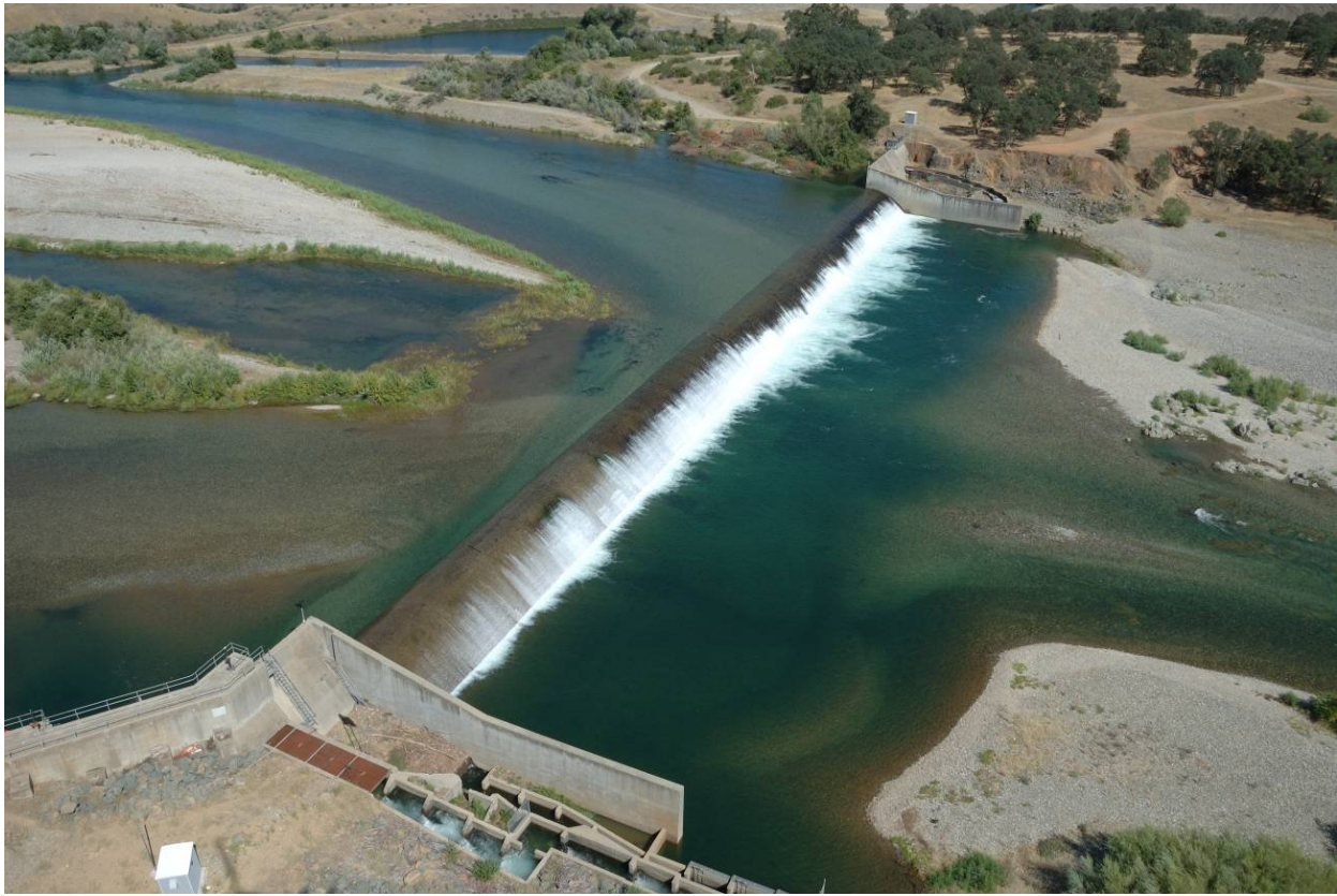
Figure 3.2-4. Daguerre Point Dam and associated north and south fish ladders.
