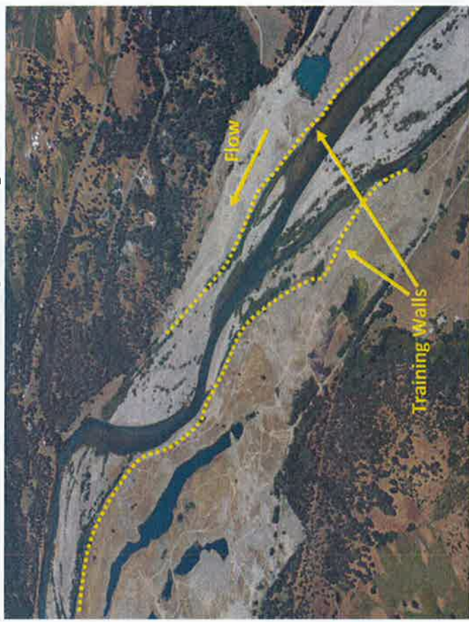
Lower Portion of Study Reach Laterally Confined by Training Walls
